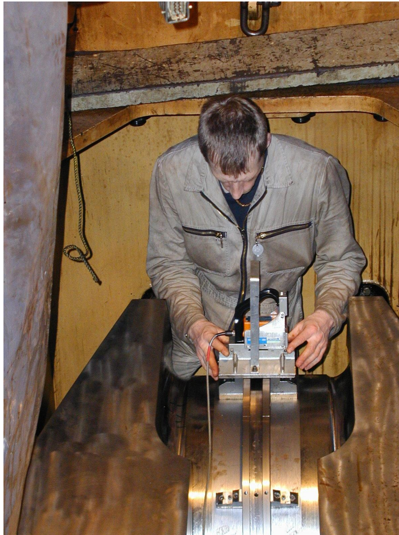
Setting a false ring to re-machine the fillet radi
